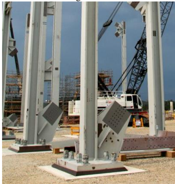
Fig. 4. Real world utilization of base plate not contemplated by current works. (Source: Author's catalogue.)
